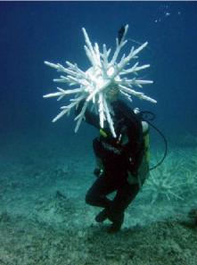
Figure 15: Diver positioning an Eco-Reefs <sup>m</sup> artificial reef module
