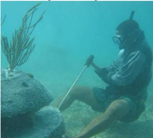
Figure 24: A diver drives a length of #5 fiberglass rebar through an anchoring tube cast into the Reef Ball. Battered rebar is driven into pre-drilled holes in the seafloor when the bottom is too hard for other techniques but vertical stability is important.
